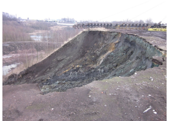
Fig. 6. Photo of the unstable zone after sliding.
