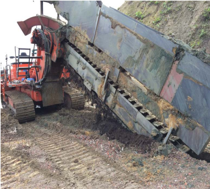
Fig. 15. Installation of the deep drainage.
