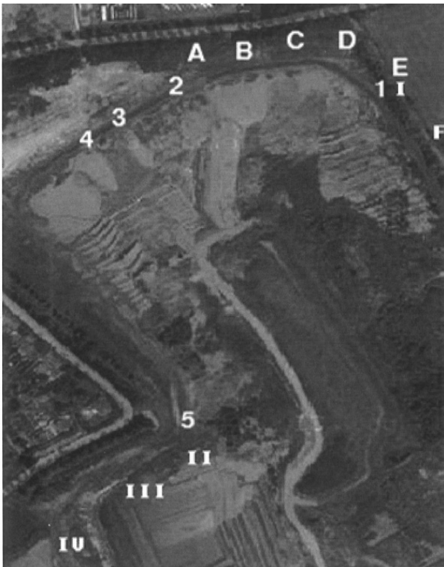
Fig. 2. Photo view of the site.
